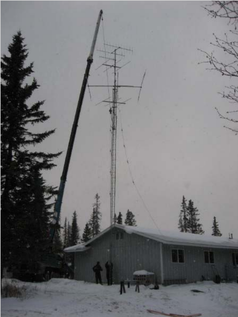
Nov. 25, 2008 – Boom Truck raises tower and sets Dish!
