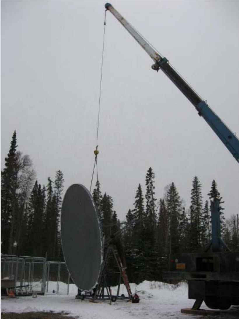
Nov. 25, 2008 – Boom Truck raises tower and sets Dish!
